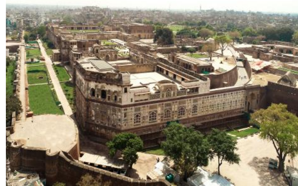
Restored western facade of the Picture Wall of Lahore Fort
